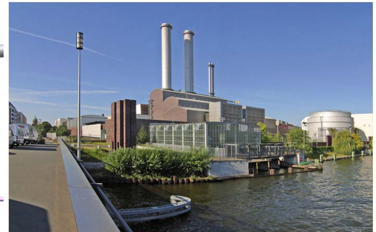
Combined heat and power plant Berlin Mitte Vattenfall Europe Berlin
