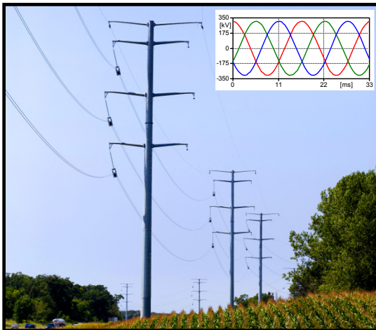
Figure 1. Transmission Line Selected for Study
