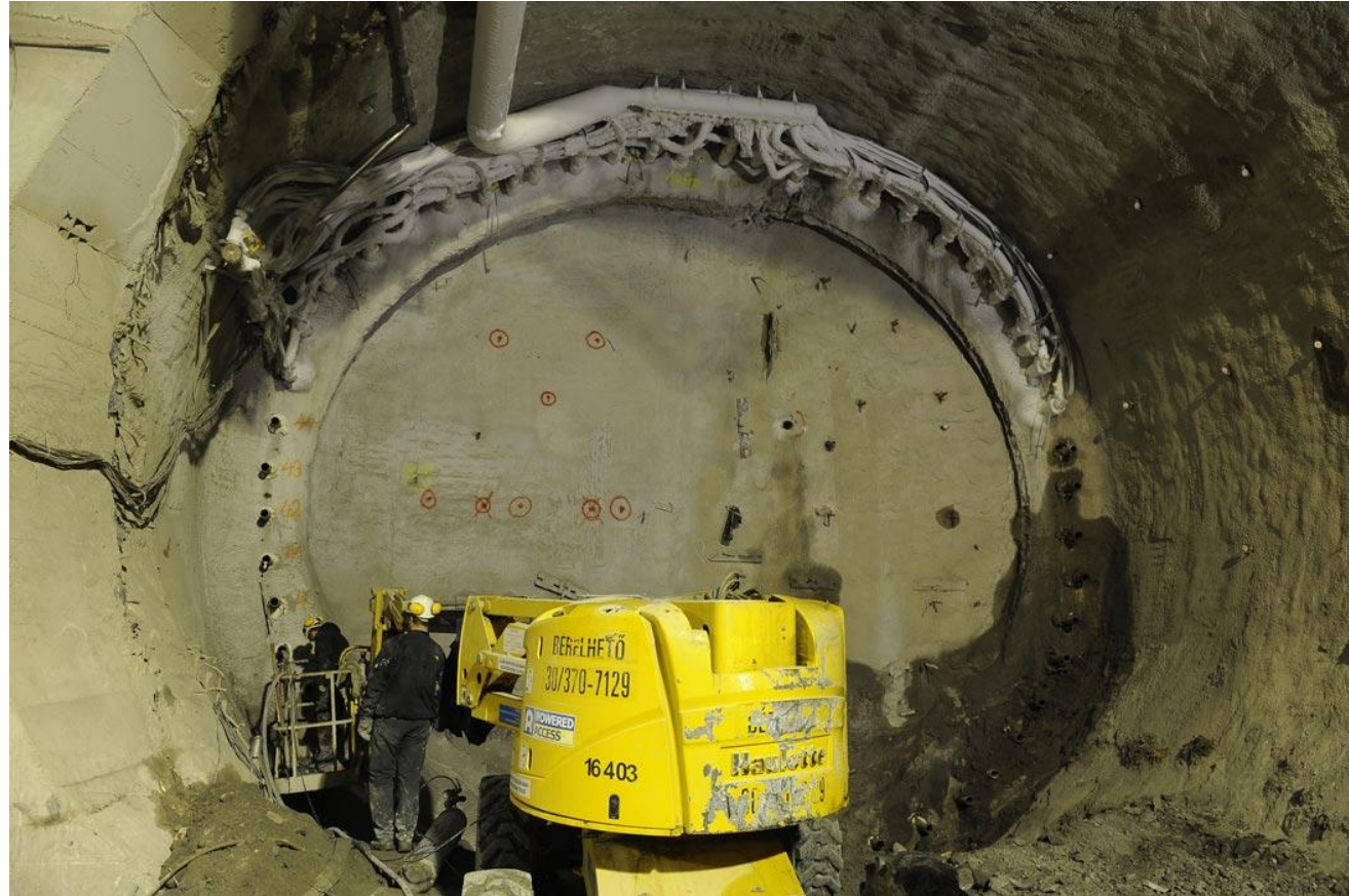
Construction of the metro line 4 in Budapest ©Tunneltalk.com
