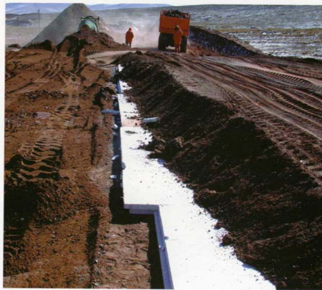
Figure 24. Scenery of thermal insulation embankment construction
