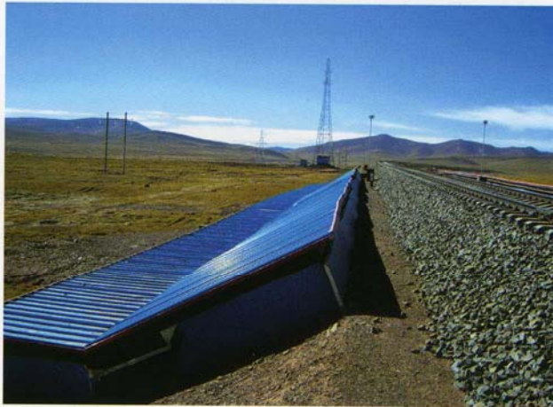
Figure 32. Scenery of sunshine shield railway embankment
