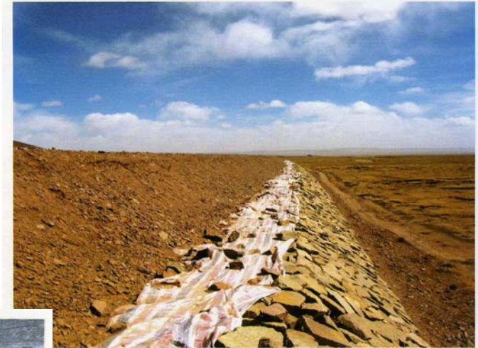
Figure 30. Scenery of air convection railway embankment
